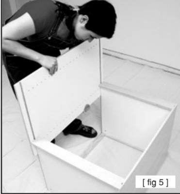
Repeat STEP 3 for the other side panel see fig. 5 and 5A. Take the corner blocks and 1/2" screws and attach to face frame and side panels (see fig. 5B and 5C) in the middle of the cabinet. (see fig. 5D)
