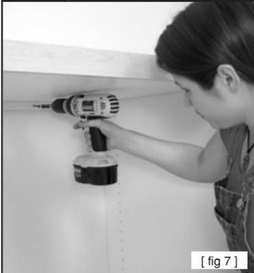
After glue is dry locate studs in wall (fig. 7A). Attach cabinet to wall using 2 1/2" screws. (See fig. 7)
