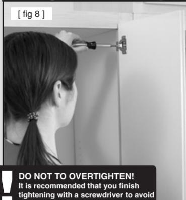
To hang doors, use the 1 1/2" silver screws. Hold door up so the door hinge hole lines up with the pre-drilled hole in the face frame. Screw in the hinge so the doors are level across the top and flush in the front. Take clear bumpers and attach as in fig. 8B, to top and bottom of doors.
